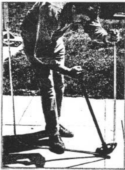
THE CANOPY FRAMING is made of electrical conduit tubing. It's bent with a hickey.
