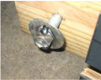
Stud with nut and washer welded to it for the slotted steel plate to slip on
