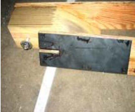
Stud with nut and washer welded to it for the slotted steel plate to slip on
